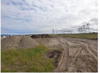
Image 8: Stockpiling of aggregate material.
