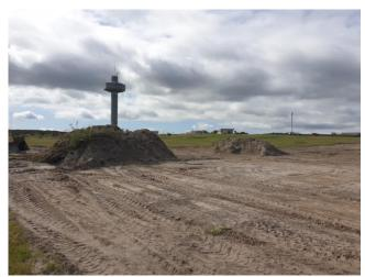
Image 4: Top layer of area to be cleared for car park extension stripped and stockpiled.
