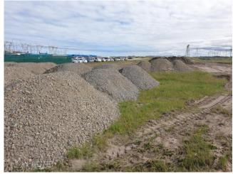
Image 7: Stockpiling of aggregate material.
